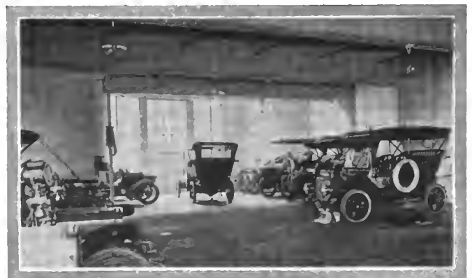
LOOKING TOWARD FRONT OF BUILDING ON SECOND FLOOR.
